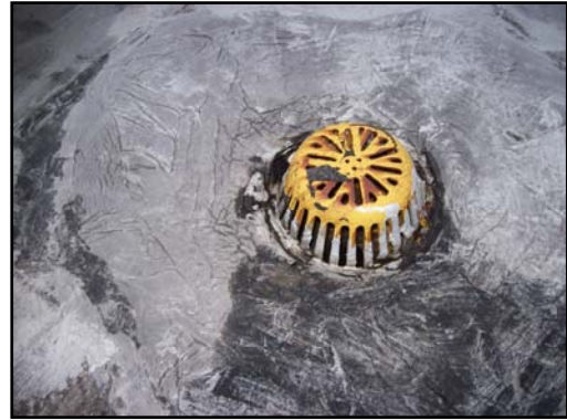
Typical roof drain.
