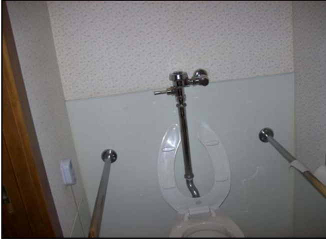
Typical resident room toilet
